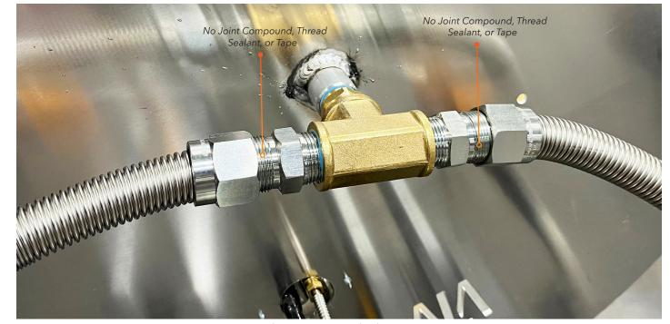
Photo 20: Connecting the Flex Lines
